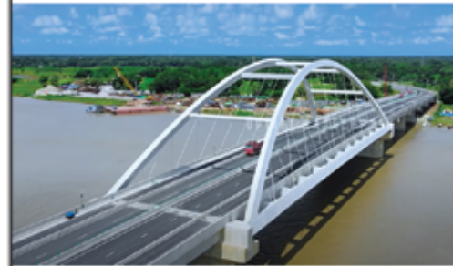
Kalna Bridge under Cross Border Road Network Improvement Project
