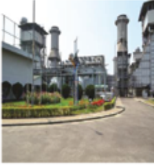
Mymensingh 210 MW Power Station
