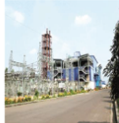
Raozan 25 MW Dual-Fuel Power Plant
