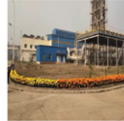
Gazipur 105 MW HFO Fired Power Plant
