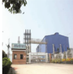
Gazipur 52 MW Dual-Fuel Power Plant
