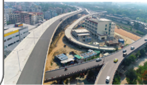
Dhaka Elevated Expressway PPP Project
